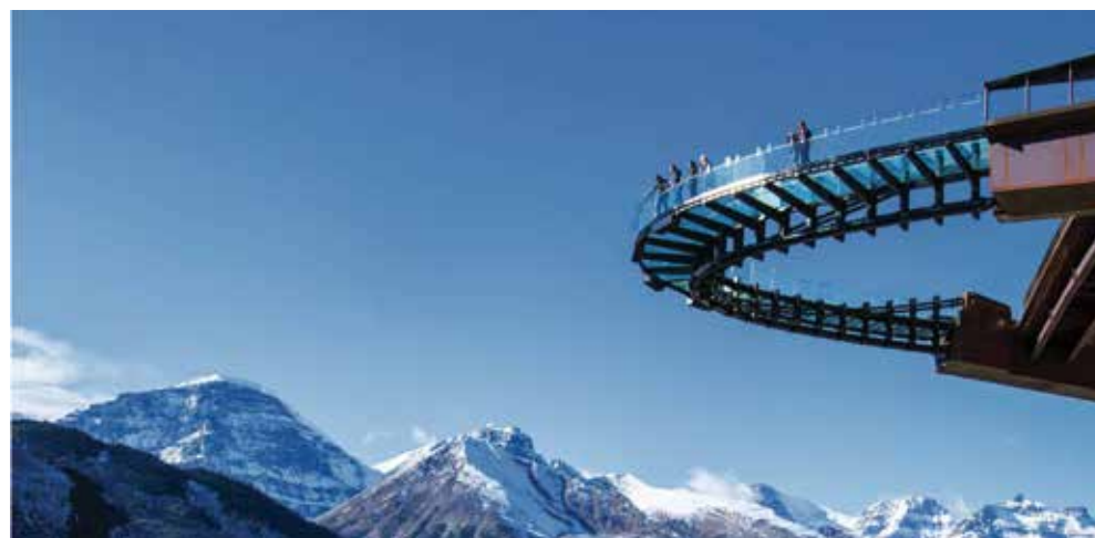
12mm Laminated Glass with 0.060 SGP Interlayer
