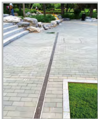
The U-Shaped Linear Drainage trench
