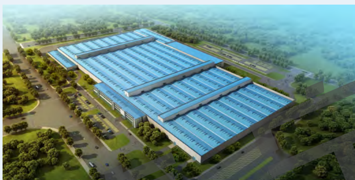
北京奔驰发动机联合厂房 New Engine Plant of Beijing Benz
