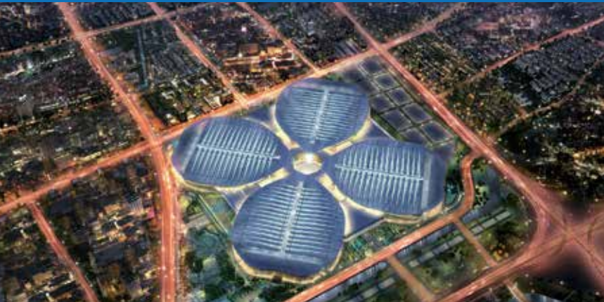
工程名称：上海虹桥商务区中国博览会展综合体 China Expo exhibition projects in Shanghai Hongqiao business district 屋面面积/Roof area：420000m 2
