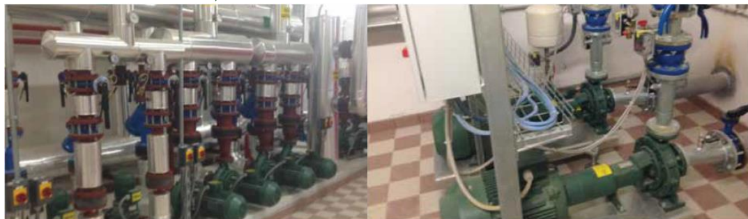
科特迪瓦国家银行消防系统 FIRE-FIGHTING SYSTEM EN12845 FOR THE NATIONAL BANK OF ABIDJAN (IVORY COAST)
